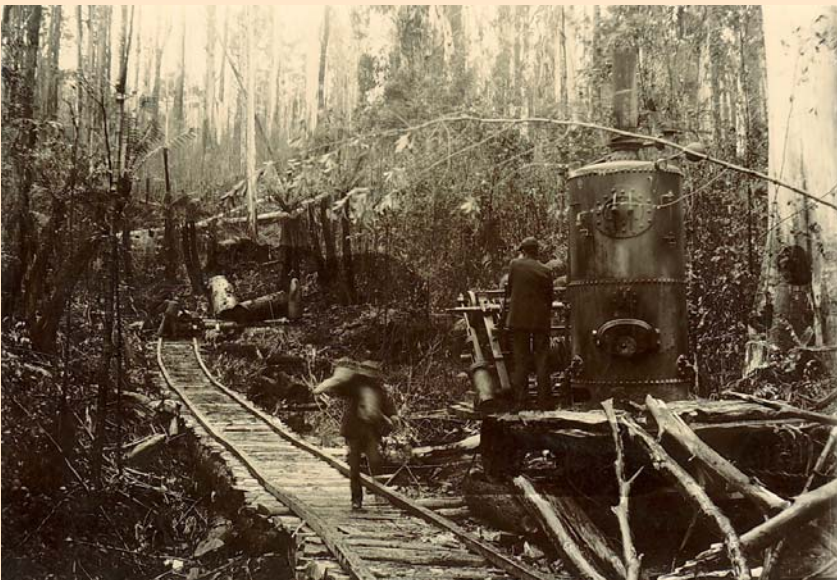
A Timber tramline. Photograph by P. King, courtesy of DSE.
